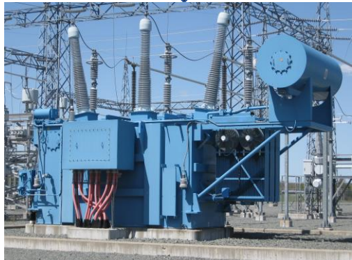
Transformer to reduce voltage for local distribution
