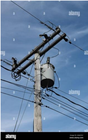
Transformer to reduce voltage for local distribution
