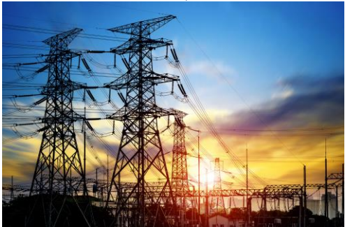
Long Lines To Local Utility
